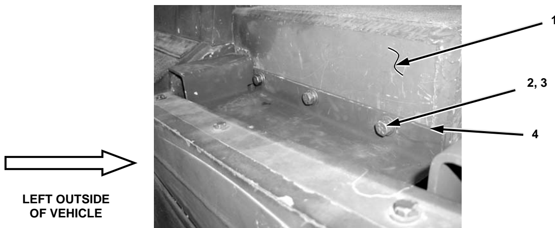
Figure 2-20. Coolant Umbilical Guard Installation.
